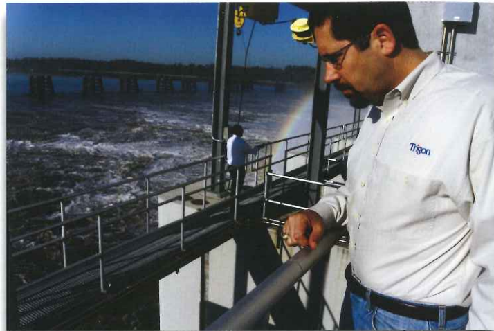
Greg is on site at a flood protection structure during operation near New Orleans, Louisiana.
